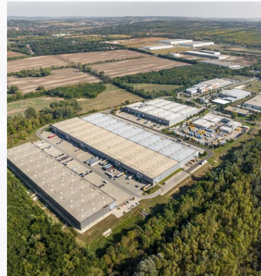
EAST GATE BUSINESS PARK
