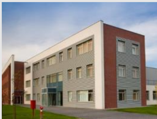
East Gate Business Park
